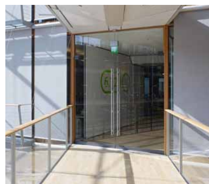
The glass doors leading to the individual storeys are equipped with floor springs from DORMA.
